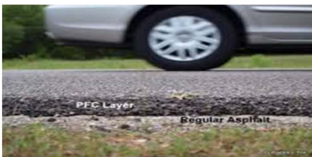
Fig. 1: PFC (OGFC) layer laid over the regular asphaltic layer.[27]
