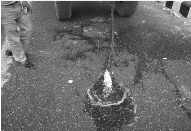
Fig. 5: Water from a tanker hose penetrating directly porous pavement [21].
