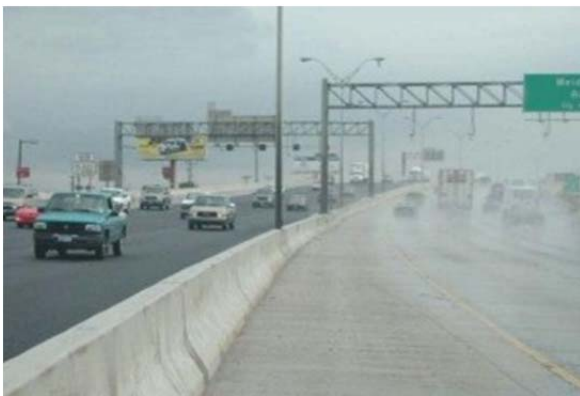
Fig. 2: OGFC surfacing on left lane (reduced splash and spray) and right lane without OGFC [28].
